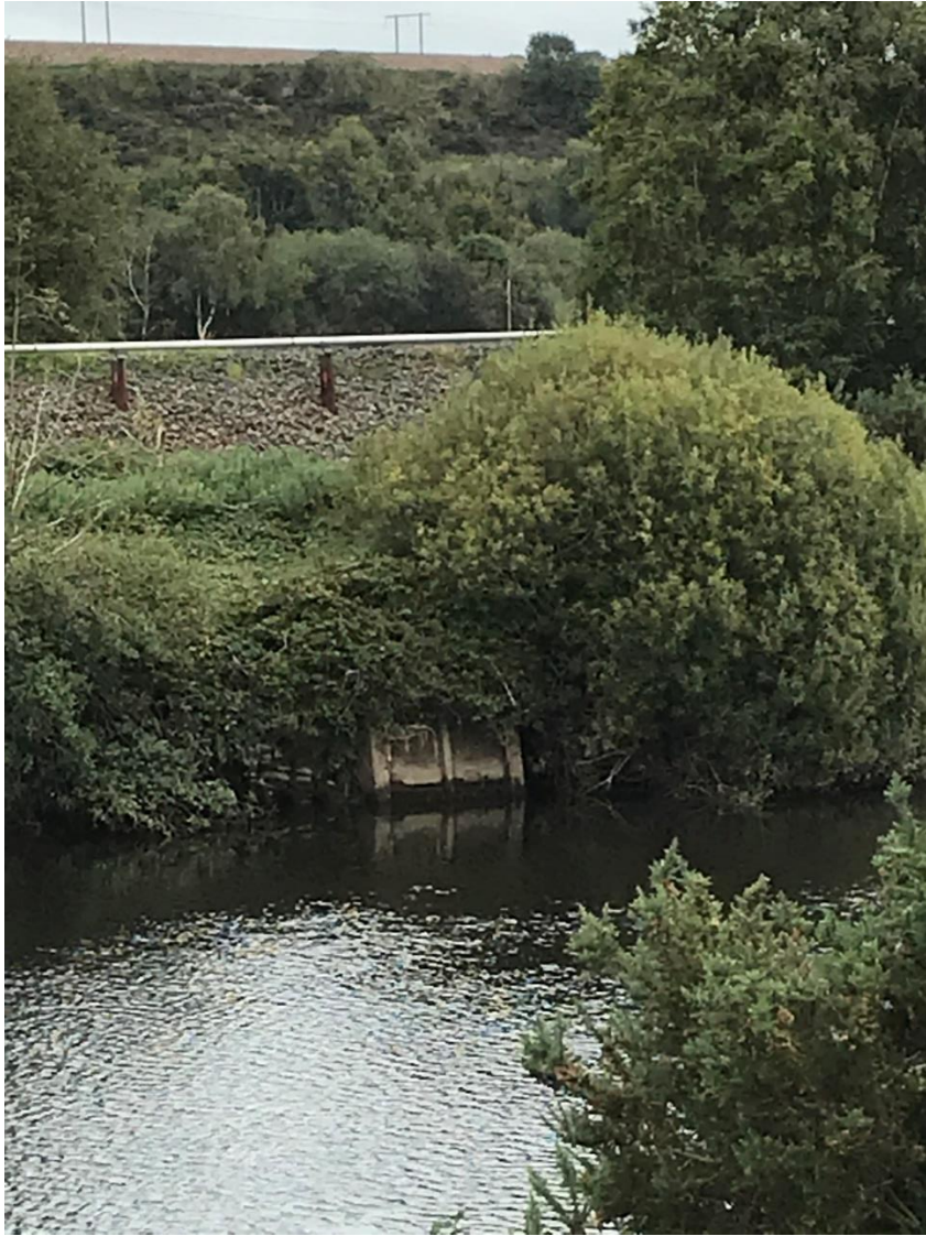
Flap vale from opposite side of the embankment from the pond
