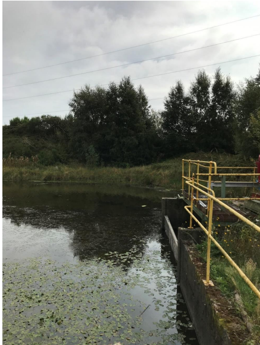
Pond and intake structure with trash screen
