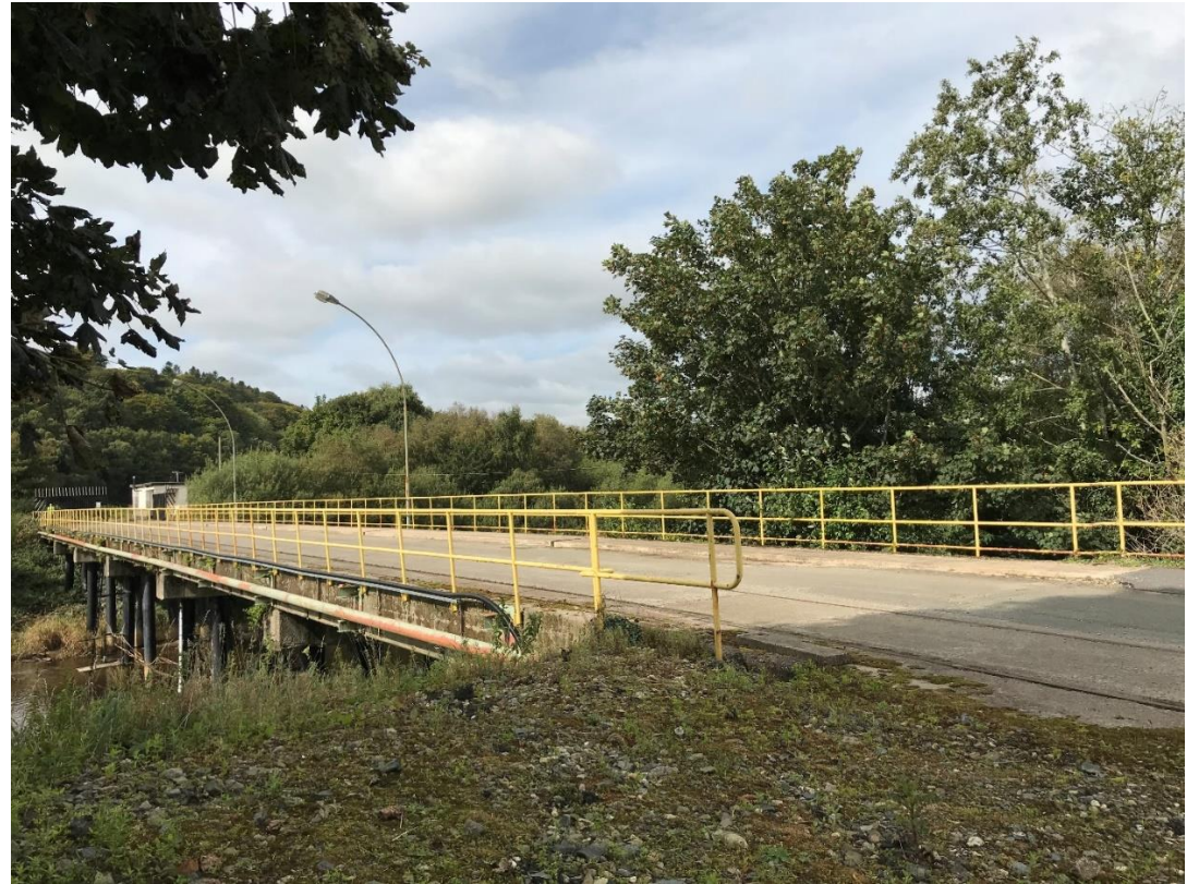
Access track road bridge
