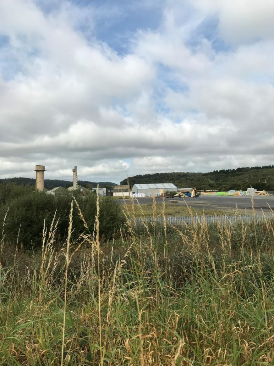
Looking across the data centre site from embankment to the east
