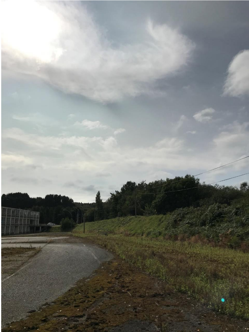
Western side embankment looking south
