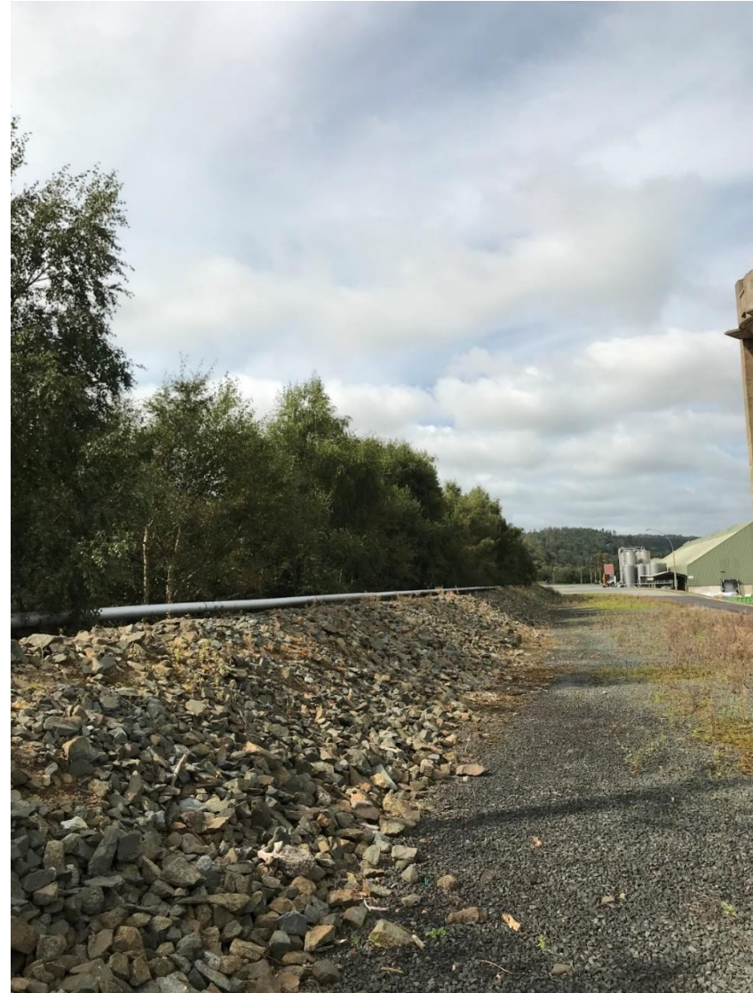
Embankment along southern side of site
